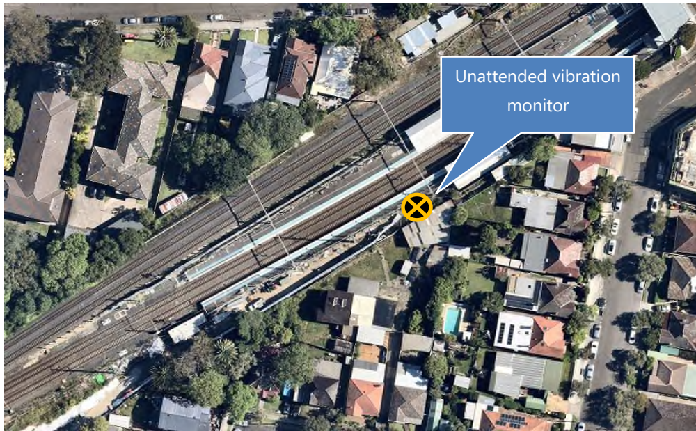
Figure 2-1: Vibration monitoring location
