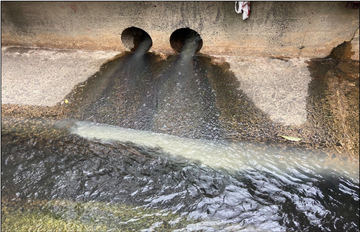
Photograph 7. High flow stormwater observed from the downstream discharge point WP2-DP2 which were located within the rail corridor and immediately upstream / south from WP2 during the monitoring event – approximately 2:30 pm 22 February 2023 (at the time of sampling).
